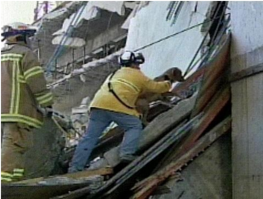
T-2 Chemical Plant Explosion
