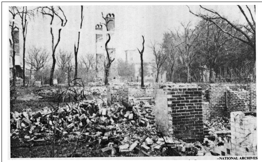
Brick chimneys remain along Forsyth Street after yankees burned the area.
